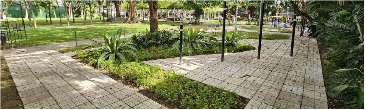
Installation of concrete pathways at Mahogany Park (Photo from DVA files)
