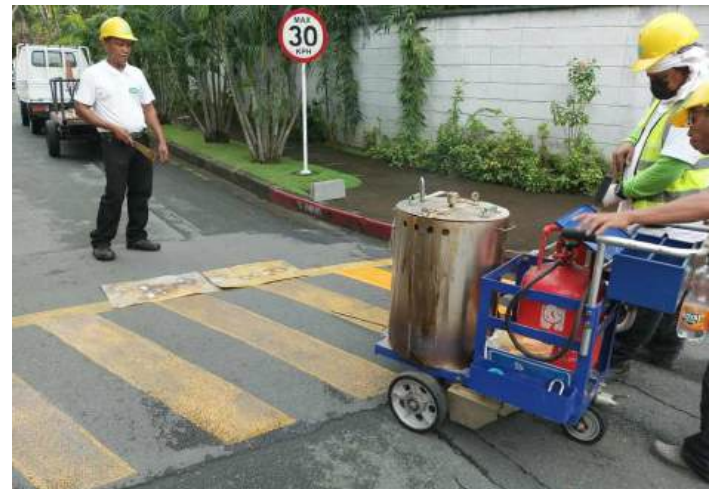
Thermoplastic paint applicator used for street markings (Photo from DVA files)
