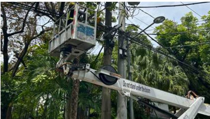
Trimming of trees to avoid contact with Meralco wires and streetlamps (Photo from DVA files)
